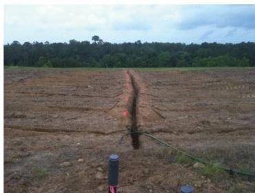
Subsurface Drip Installation. A specialized subsurface drip irrigation system was chosen for distributing leachate across the vetiver planting area.
