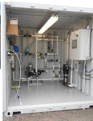
Pre-treatment and Distribution System. The engineered pre-treatment and distribution system automatically adjusts to changes in leachate production, leachate quality, and weather conditions to ensure proper operation.
