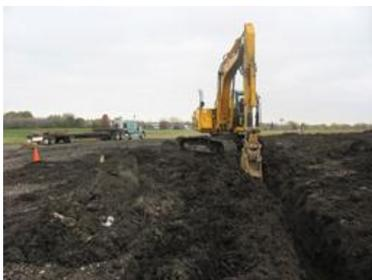
Underground Piping. Force mains are installed to convey leachate to the vetiver planting area.
